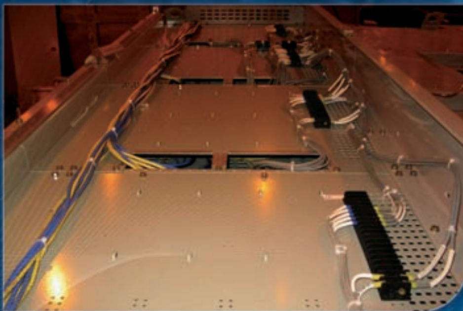
Above: Traditional switchgear wiring. Right: Entellisys' greatly reduced wiring means many fewer terminations and faster, easier installations.
