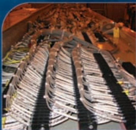
Above: Traditional switchgear wiring. Right: Entellisys' greatly reduced wiring means many fewer terminations and faster, easier installations.
